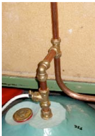
Hot tee without sleeving and insulation, before they are added
