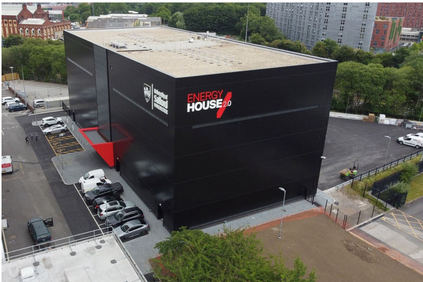
Salford's Energy House can create snow, rain, winds and temperatures from -20^{\circ}\text{C} to +40^{\circ}\text{C} to test full size house
